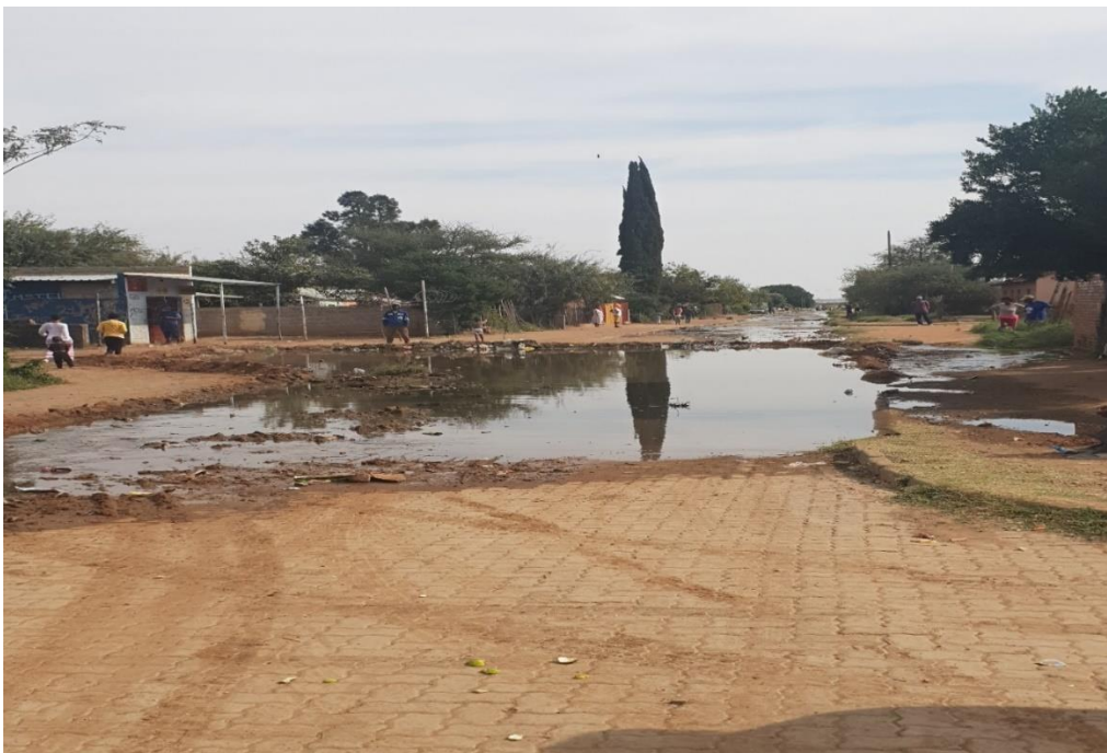
Picture 3: Raw sewerage flowing in streets in Roodepan (Roodepan CPF)
