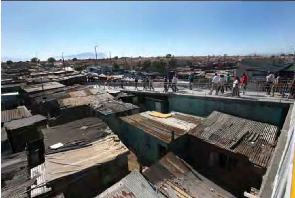
Photo 8: The inspection in loco on 21 January 2014 – crossing a railway bridge in Site C
